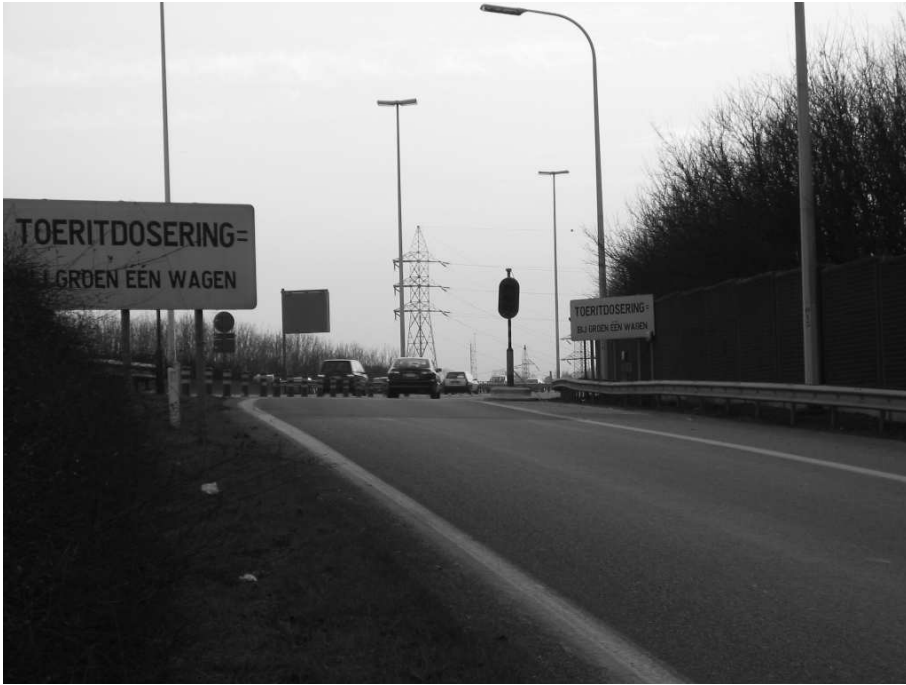
Figure 2.11: Picture of the ramp metering setup on the E314 on-ramp in Kessel-Lo, Belgium.
