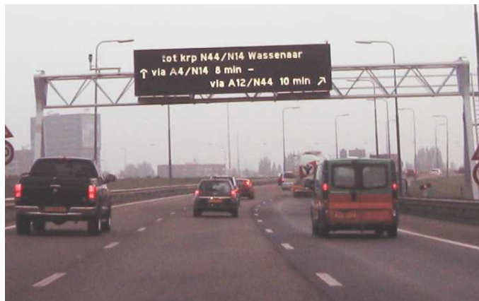
Figure 1.4: Dynamic route information panel.
