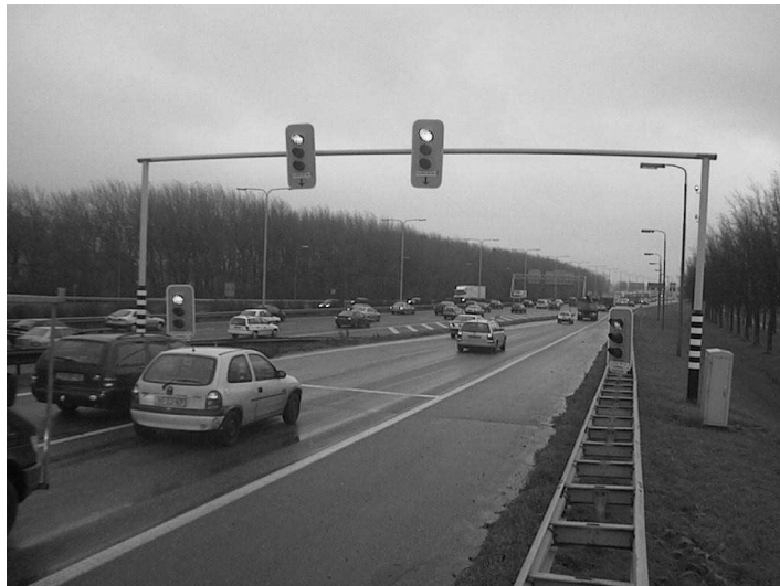
Figure: Ramp metering on the A13 highway in Delft-Zuid.
