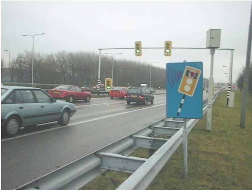
Figure 25: Ramp metering on the A13 highway in Delft-Zuid.
