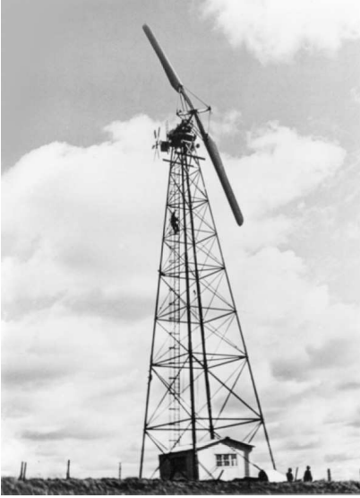
(a) F. L. Smith wind turbine (1941) with a rotor diameter of 17.5m and rated power of 50kW.
