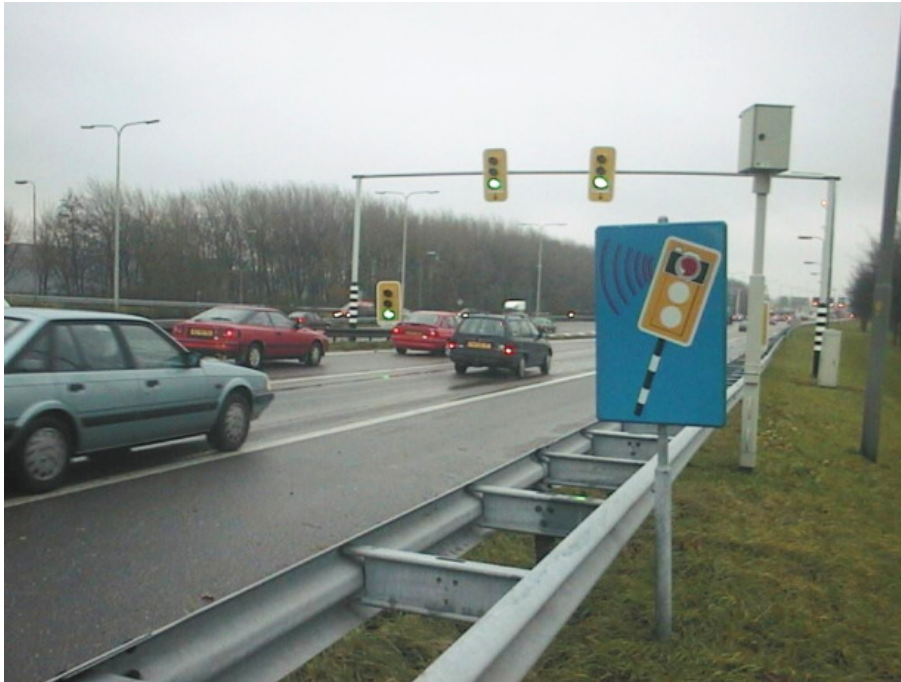
Figure 7: Ramp metering at the freeway A13 in Delft, The Netherlands. One car may pass per green phase. To prevent red-light running the control is enforced.
