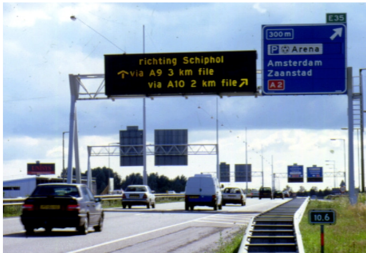
Figure 9: A route guidance system in The Netherlands showing traffic jams lengths on alternative routes to Schiphol Airport. (Photo courtesy of Peek Traffic B.V.)
