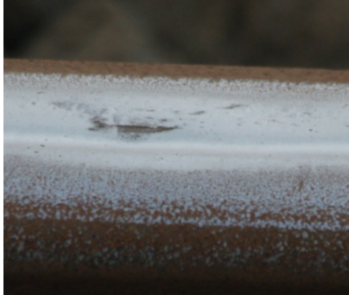
(a) Picture of the defect
