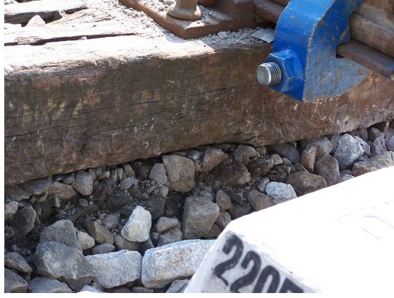
Figure 1: Severely wore ballast stones under an old sleeper. Compared with the new ballast stones nearby with sharp edges, the wore ballast stones have become rounded in shape and covered by dusts. This problem is called the "foul" of the ballast, meaning that the ballast stones have been crushed, provide less drainage, move less and have less elasticity, leading to a reduction in their friction dissipation.
