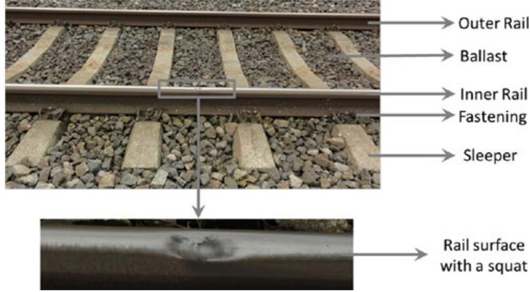
Figure 3: A severe squat on the rail surface.
