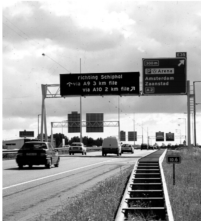
Figure 2: Dynamic route information panel. (Photo courtesy of Peek Traffic B.V.)
