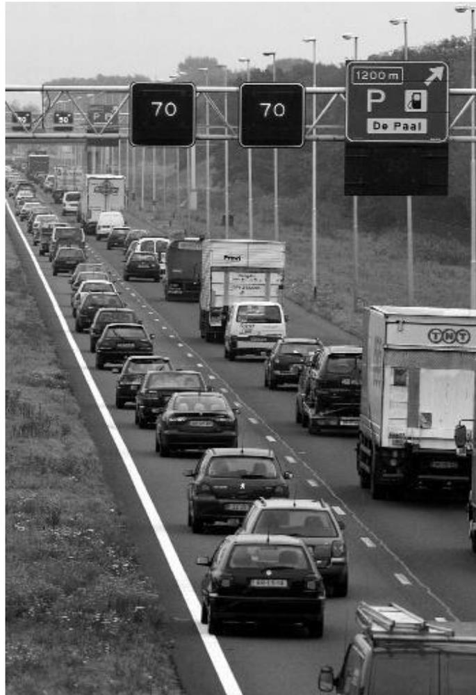
*Figure 2.3: A variable speed limit gantry on the A1 freeway in The Netherlands.*
